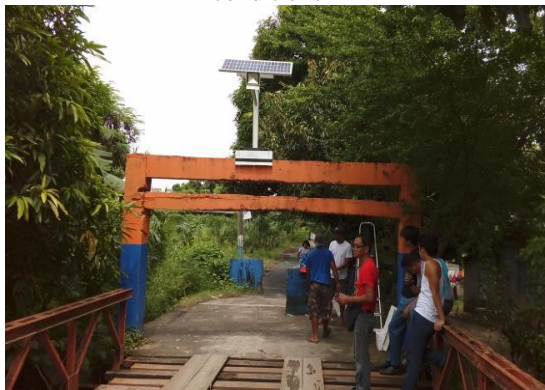
(c) Final testing and fastening of installed units to concrete posts
